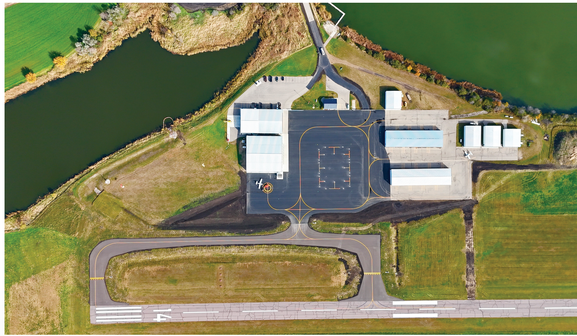
Aerial view showing the apron expansion and Taxiway Alpha, and surrounding landscape.
