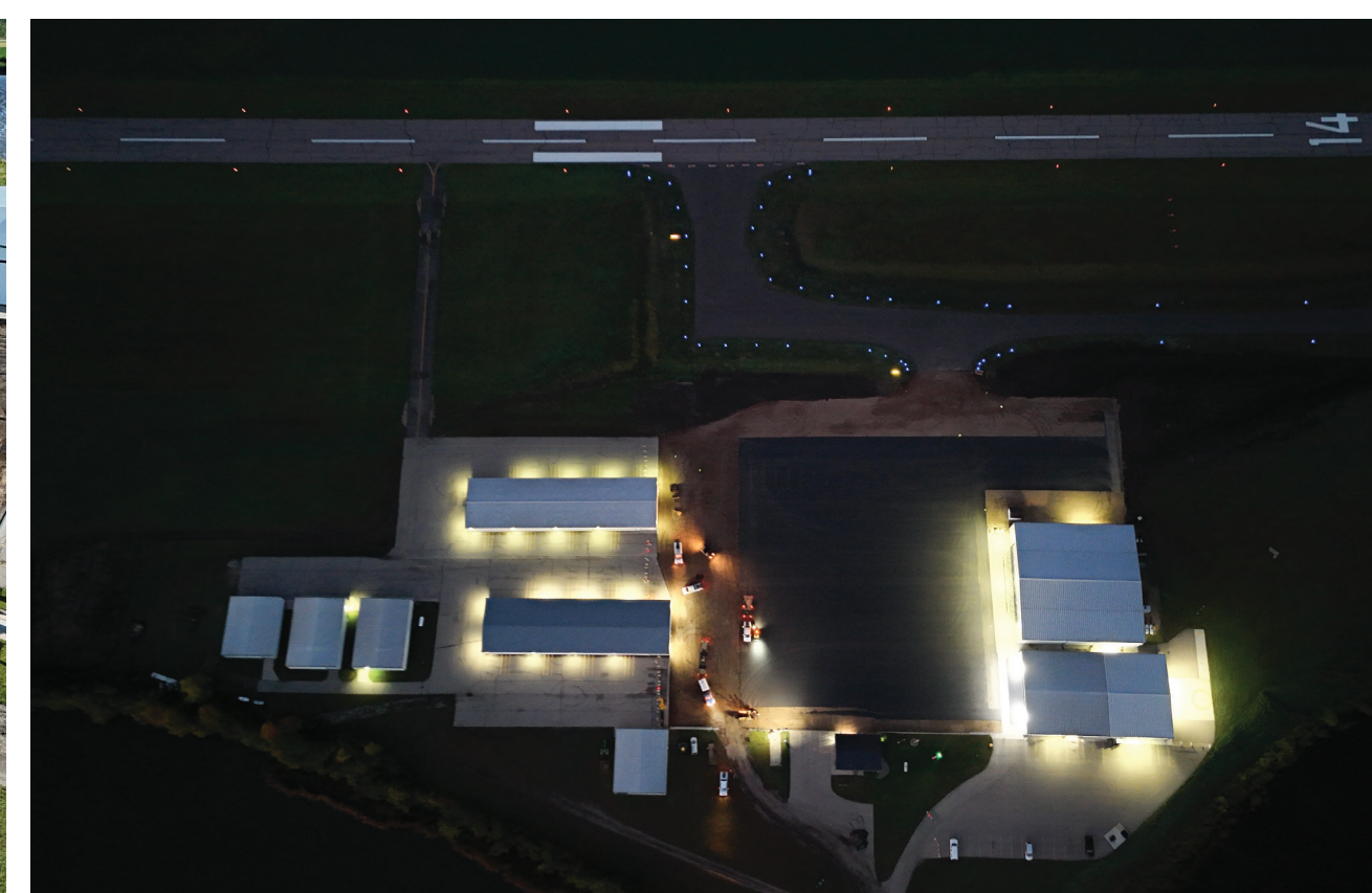
LED lighting along Taxiway Alpha enhances nighttime safety and visibility (under construction).
