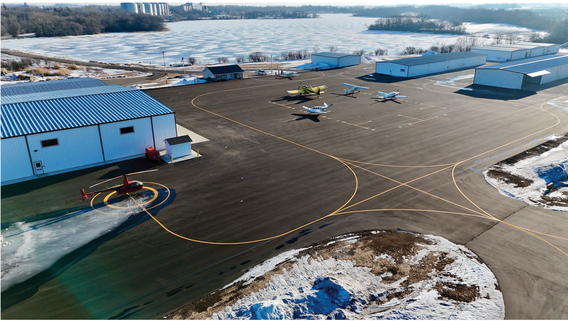
Completed apron provides greater capacity and smoother, safer ground operations.
